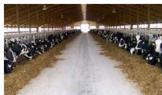
Good ventilated housing structure
